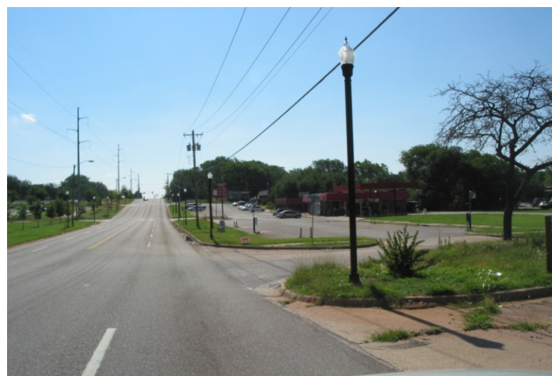
Existing Conditions: NE 8th Street Looking East
